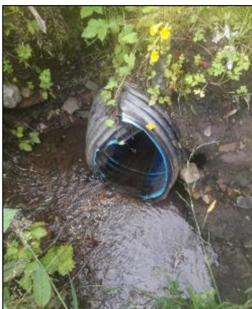
Figure 12: 'Culvert Inlet 1' captured during CCTV survey operations on 30/06/2020
