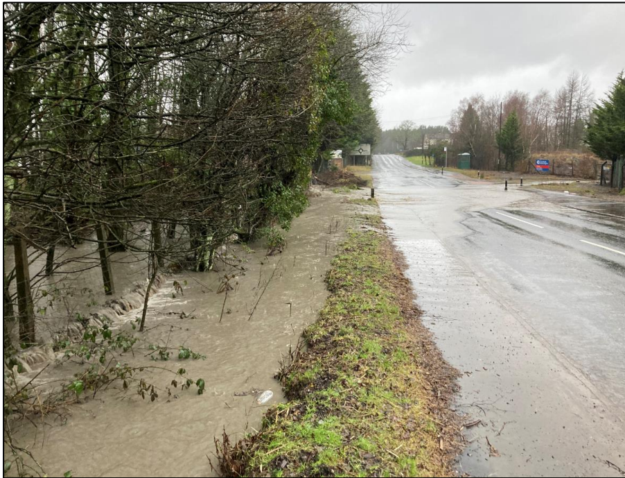
Figure 17: Surface water flooding to the A4061 Rhigos Road caused by surcharging culvert inlets associated to sub-catchment TIP 107A and TIP 107B (captured by RCT's Highways and Streetcare Depot on 16 th February 2020)
