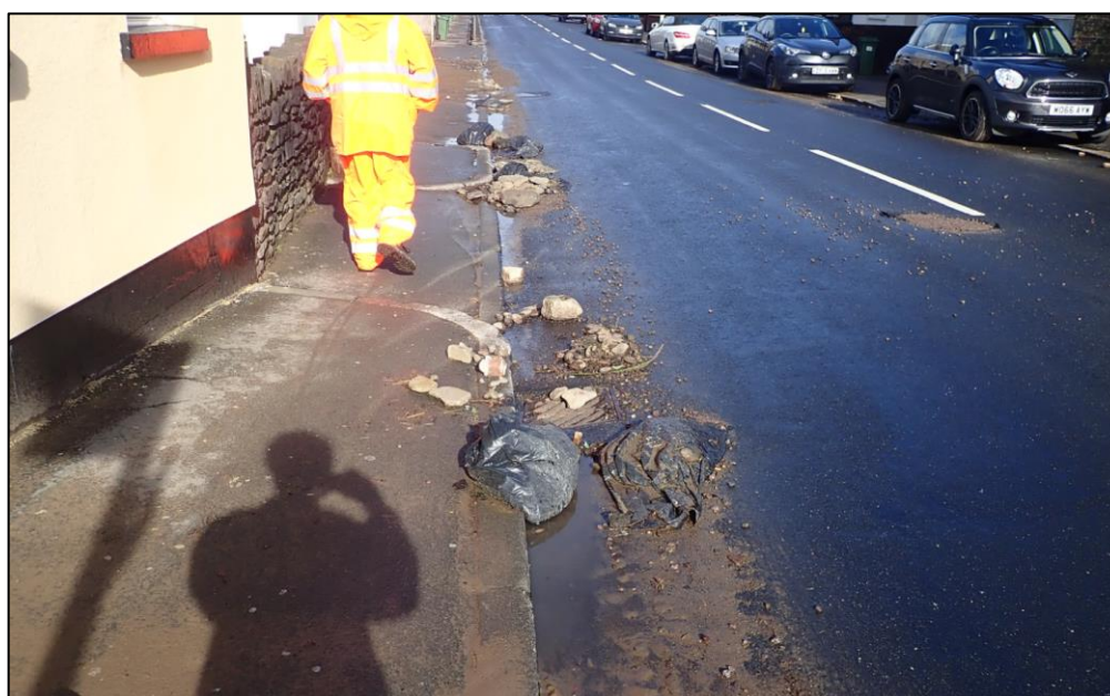
Figure 31: Debris left after the storm event at Pontshonnorton Road (captured by FRM officers on 17th February 2020)
