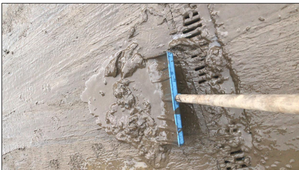
Figure 12: Photo shows deposits of mud blocking the surface water drainage infrastructure at Park Lane following the flooding during Storm Dennis (image provided by resident)
