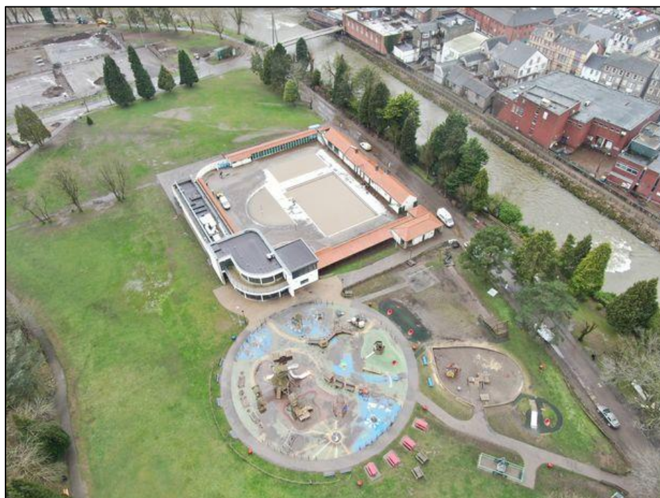
Figure 8: Image showing the flood damage to the National Lido of Wales at Ynysangharad Park following Storm Dennis (Image: Jonathan Lawrence/WalesOnline)
