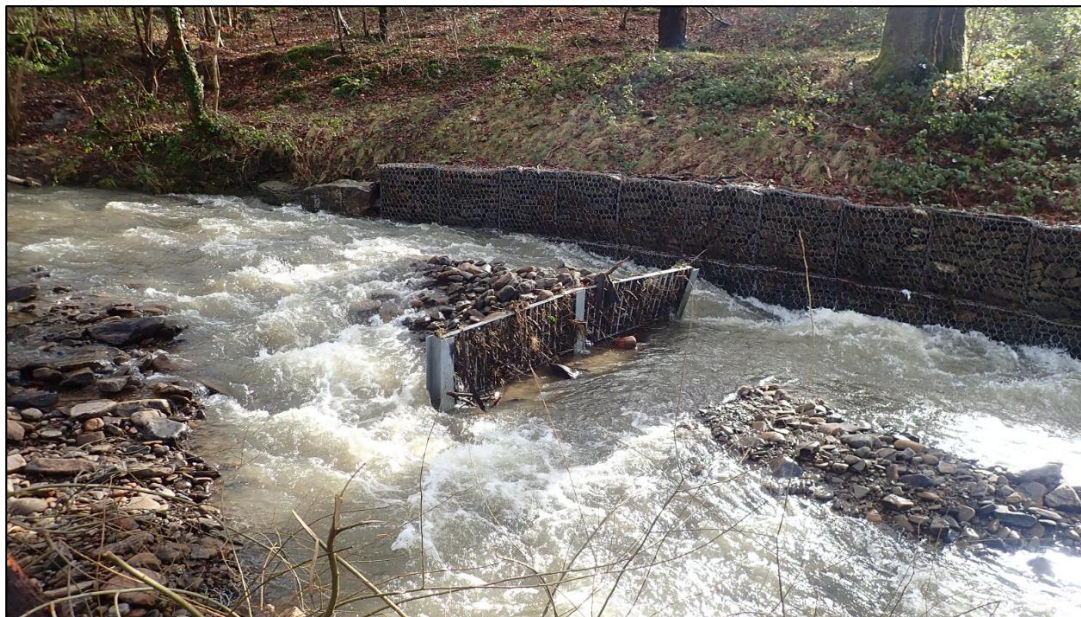
Figure 23: Second upstream debris screen in the Nant Cae Dudwg watercourse (captured by RCT's Flood Risk Management team on 17 th February 2020)
