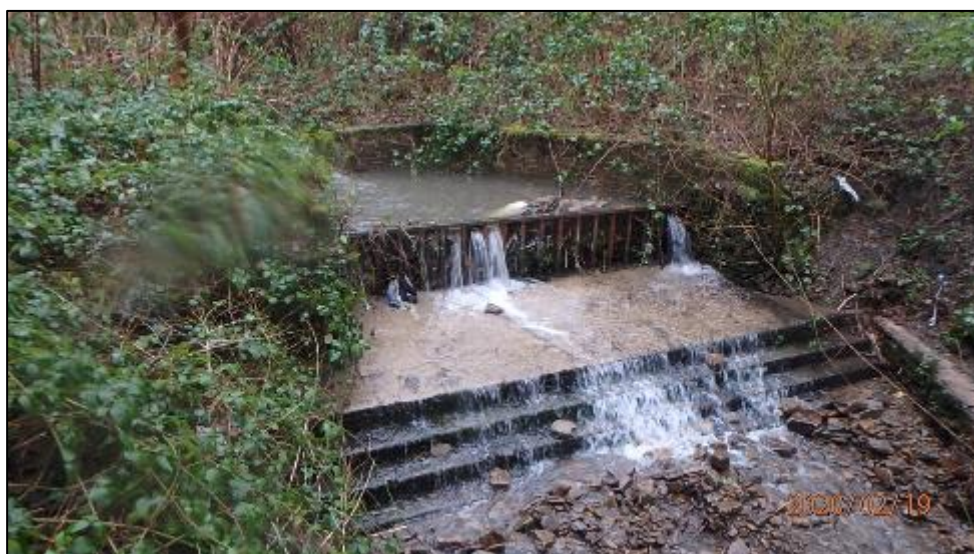
Figure 22: Photo of debris deposition behind the upper debris screen of the Nant Coedcaetylleforest ordinary watercourse (captured by RCT's Flood Risk Management team on 19/02/2020)
