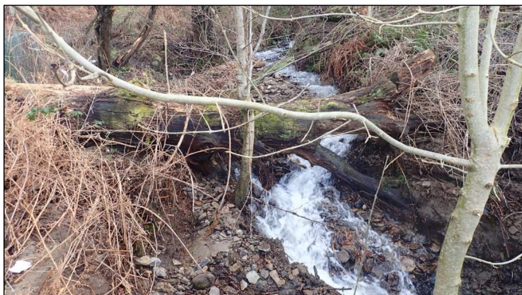
Figure 29: Tree collapse in the unnamed ordinary watercourse to the rear of Heol Mynydd (captured by FRM officers on 17 th February 2020)
