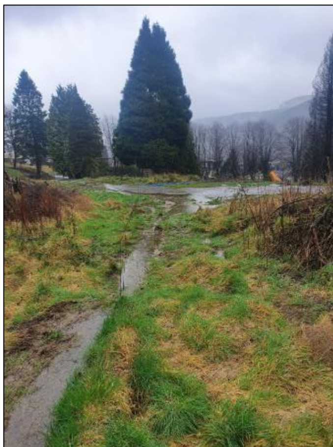
Figure 8: Overland runoff originating from 'Culvert Inlet 4' flowing along the track road to the rear of Dumfries Street (image captured by RCT's Flood Risk Management team post event on 18 th February 2020)
