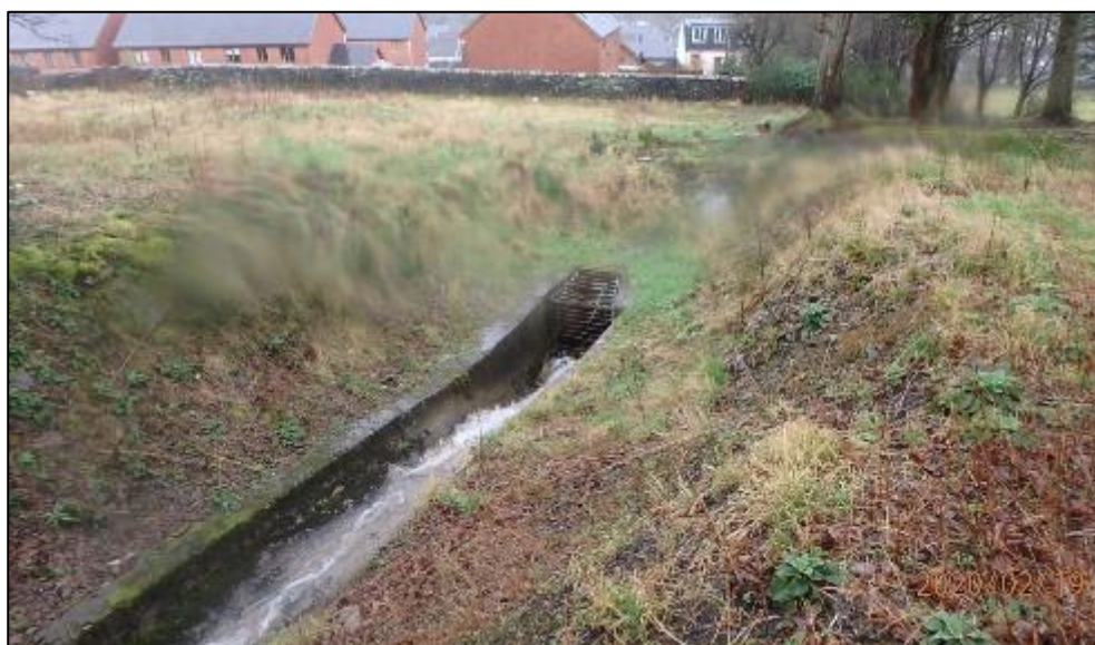
Figure 24: Culvert inlet at Area 2 which conveys the Nant Coedcaetylleforest ordinary watercourse towards Area 3 (captured by RCT's Flood Risk Management team on 19/02/2020)
